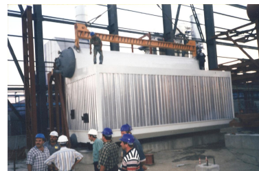
Boiler Insulation
