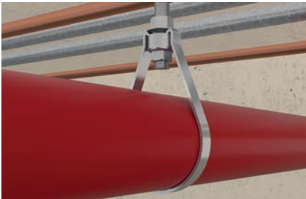
Sprinkler pipe installation
