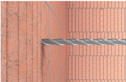
Drilling in perforated brick
