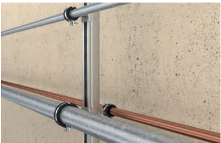
Lateral pipe mounting at channel
