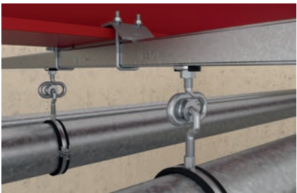
Channel fixing to steel beam
