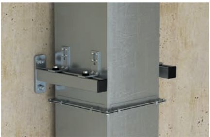
Air duct vertical installation utilising LKHS
