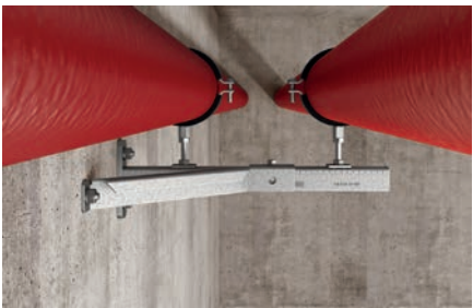
Bracing of cantilever construction
