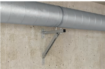
Spiral airduct on cantilever
