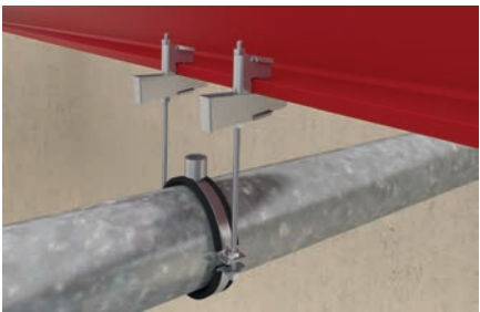
Heavy steel pipe suspended on steel beam
