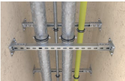
Pipe installation in escape route
