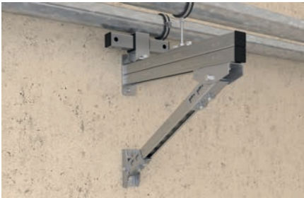
Massive bracing of cantilever arm
