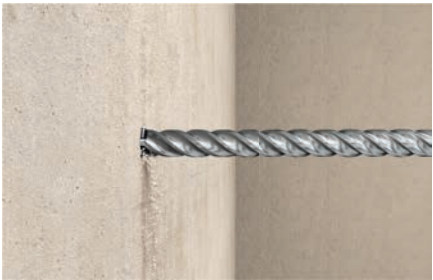
Drilling in concrete wall
