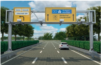
Bridges for traffic signs
