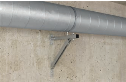
Spiral airduct on cantilever
