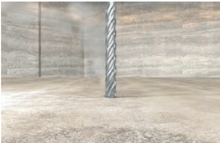
Drilling in floor plate
