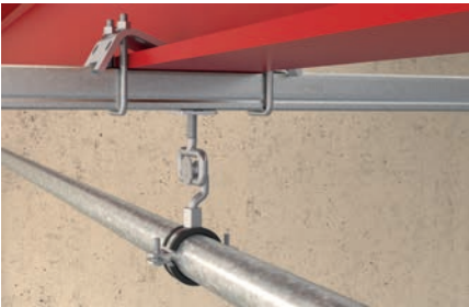
Channel to steelbeam
