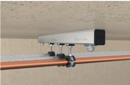
Pipe fixing at mounting channel
