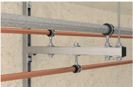
Cantilever construction with channel
