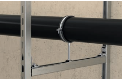
Pipe fixing on frame construction
