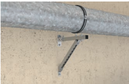
Spiral airduct on cantilever
