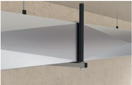
Air duct fixing with channel
