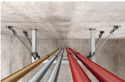
Bracing of frame construction with threaded rods
