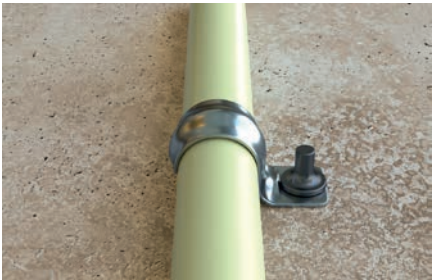
Fixing armoured conduits
