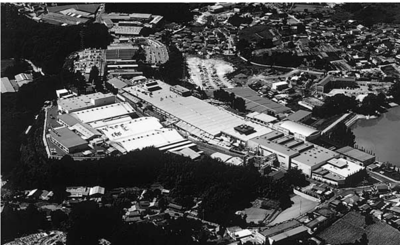
KITZ Nagasaka Plant, Japan
